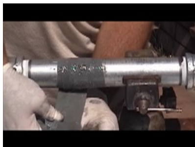
2. Apply Wrap Repair
